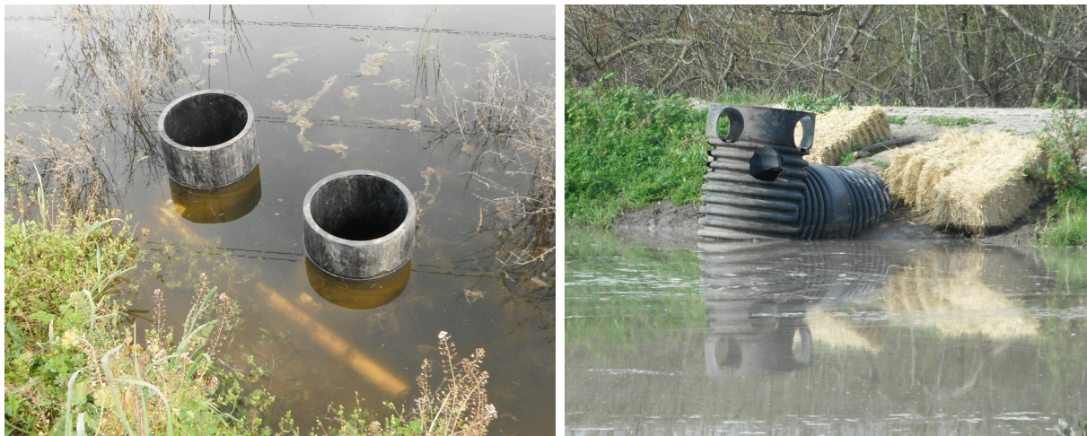
FIGURE 3. CULVERTS INSTALLED AT SOUTH FINGER MITIGATION SITE FOR WATER CONTROL. LEFT PANEL IS AT THE WEST END OF THE SITE WHERE IT DUMPS INTO MORO COJO SLOUGH. RIGHT PANEL IS AT THE SEDIMENT BASIN ON THE EAST END OF THE SITE.
